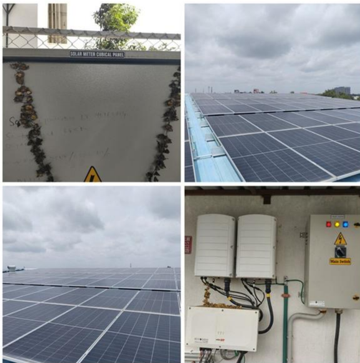
Figure 8-2: SRTPV Installed at College
