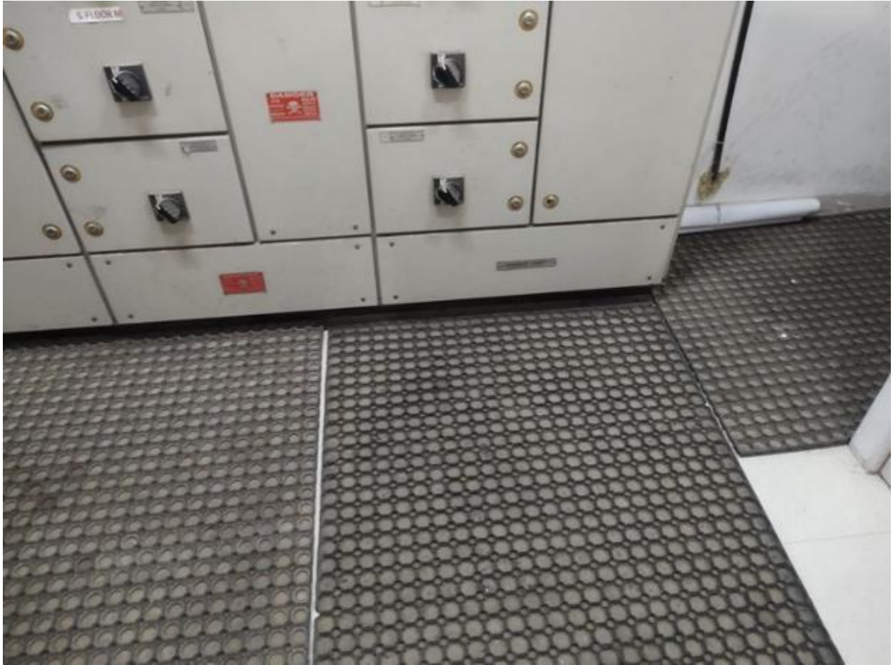
Figure 5-14: Electrical safety mats near electrical panel
