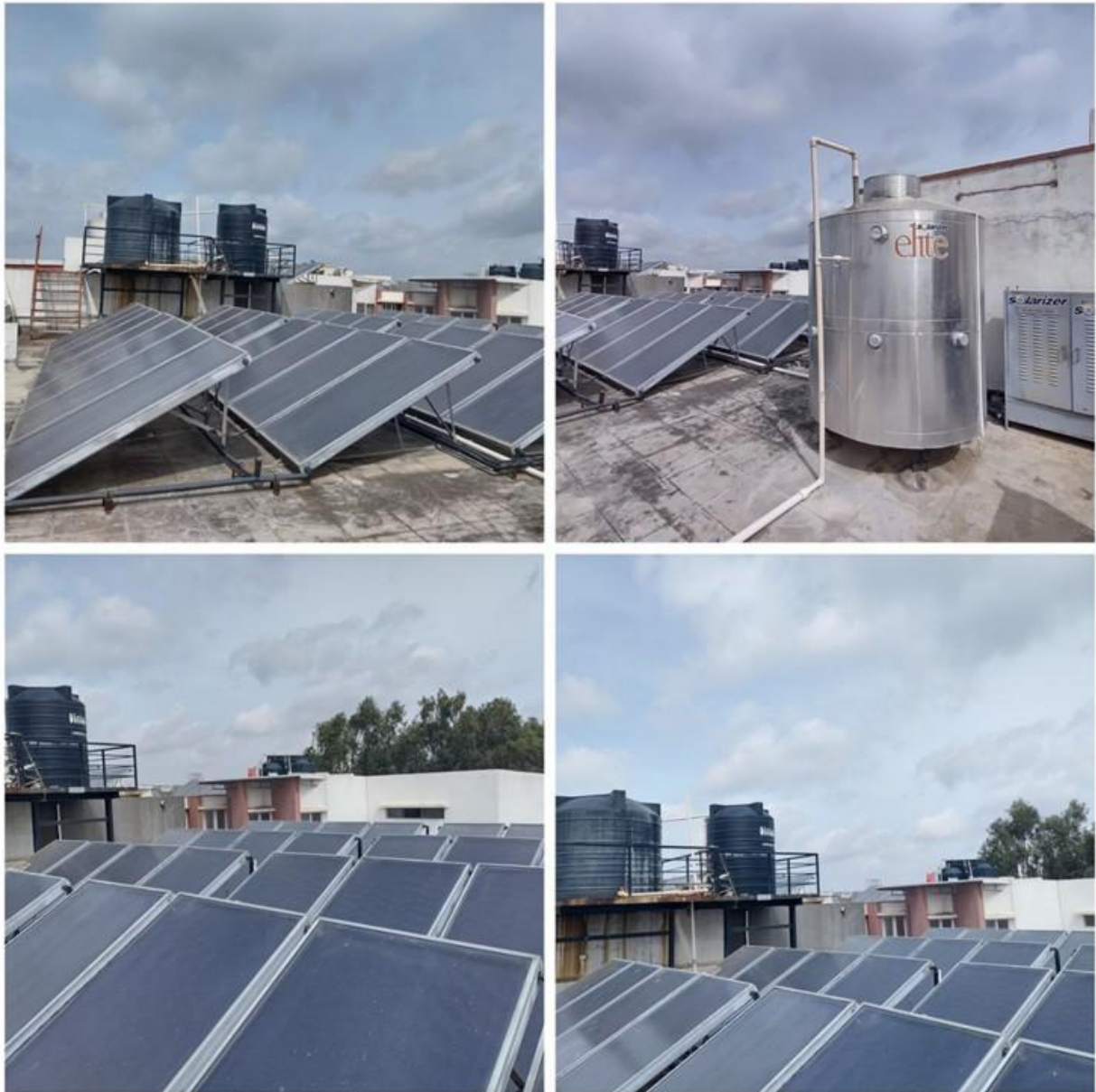
Figure 5-11: Use of Solar Water Heater
