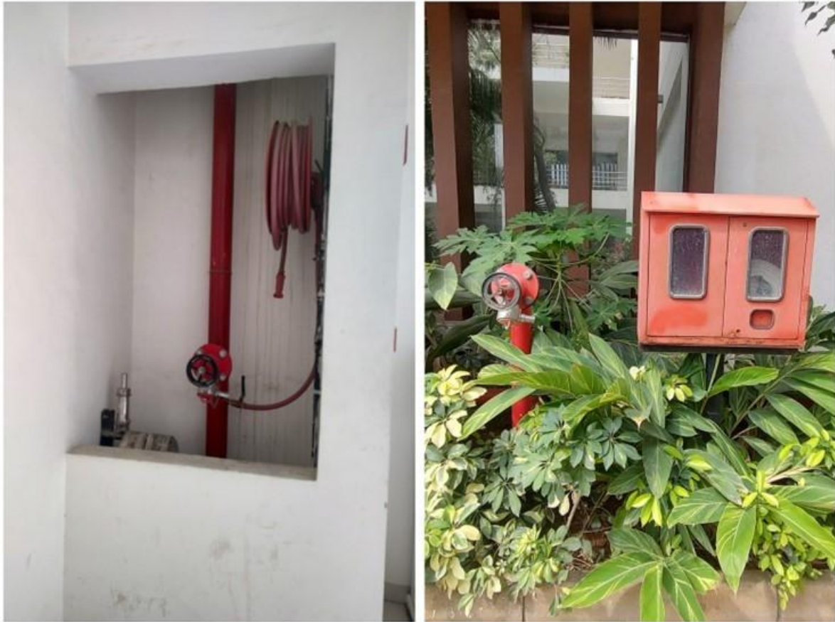
Figure 3-2: Fire hydrant system
