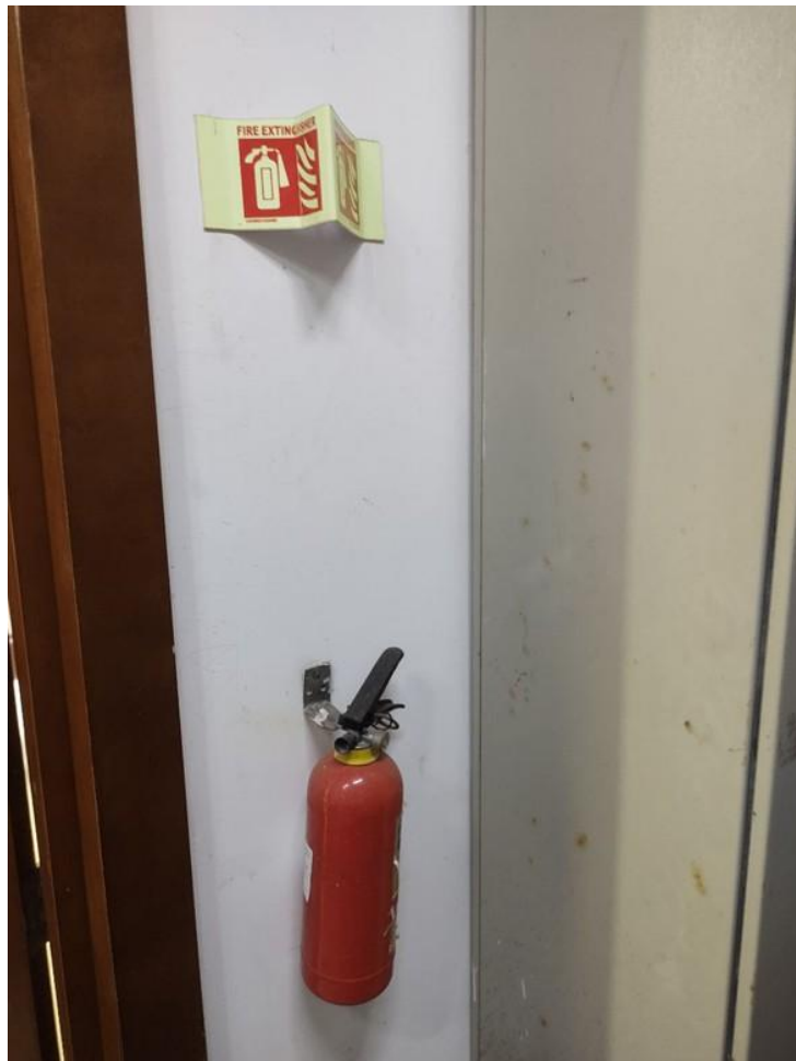
Figure 3-1: Fire Extinguisher installed in the floors
