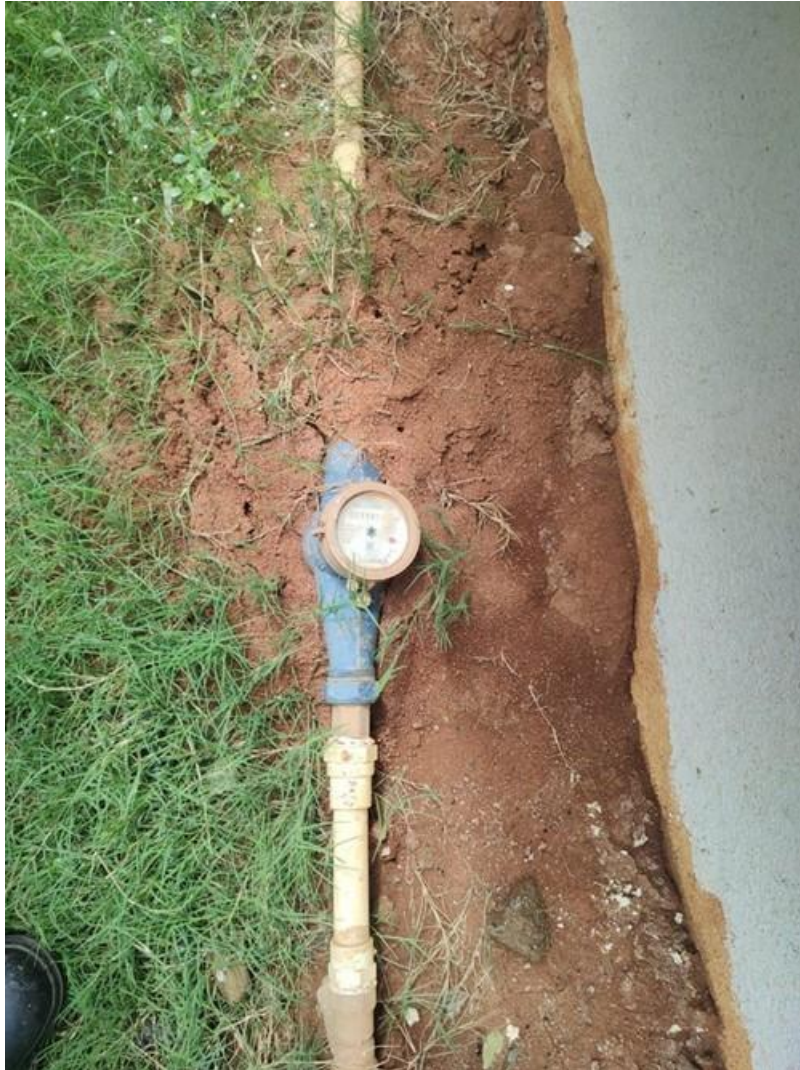
Figure 4-7: Water flow meter
