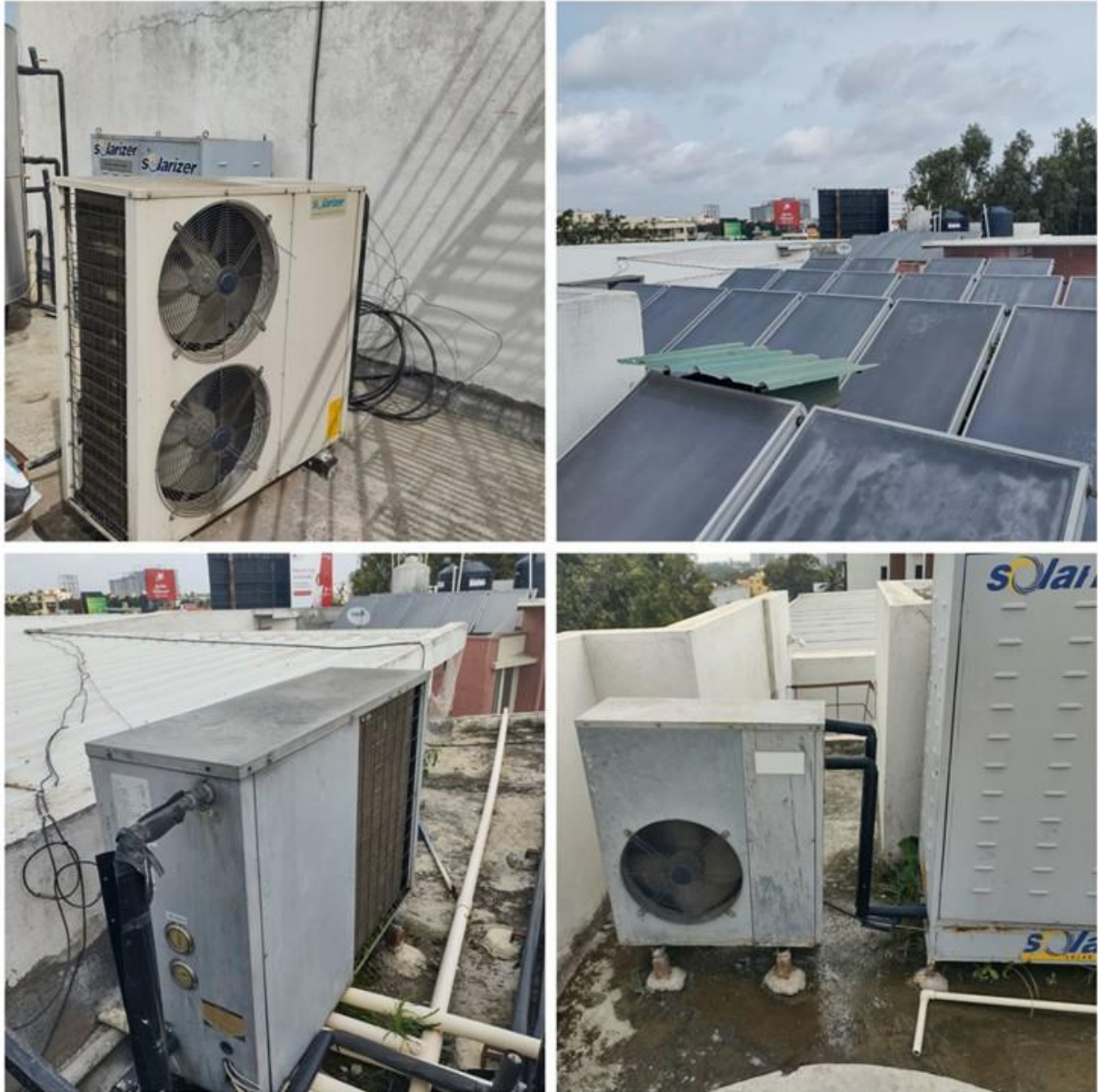
Figure 5-10: Integrated recirculation type -Hot water system
