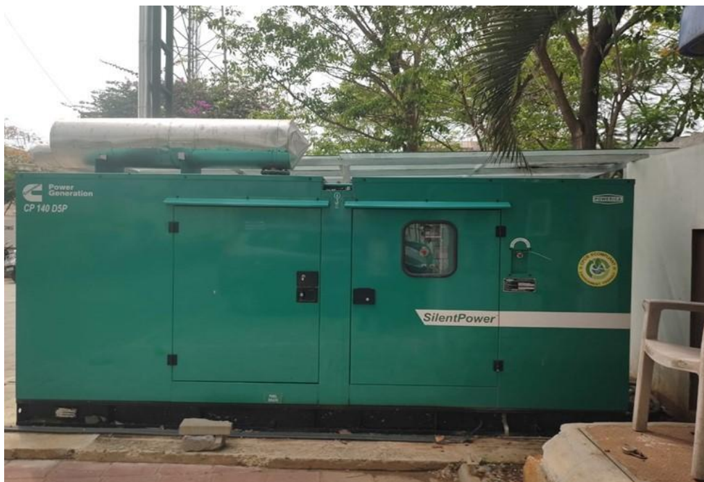
Figure 5-3: Diesel Generator (DG) sets
